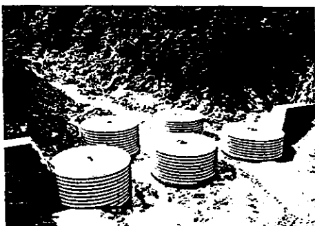
Photo 2-3. Completed Yotagiri Steel Cell Dam
